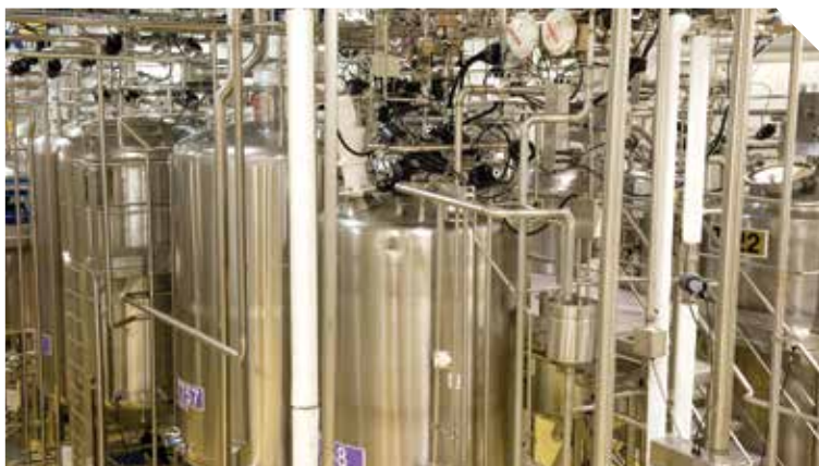
Overview of buffer preparation vessels in Albumin manufacturing facility.
